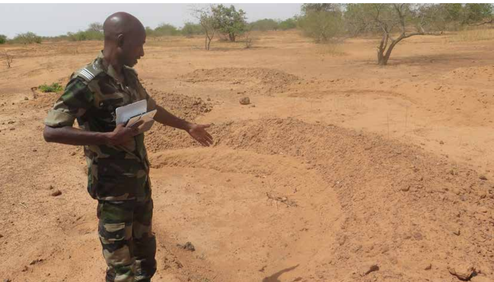
Half-moon water retention technique being implemented in Sokorbe, Niger. © Nasser Alqatami/UNCDF Niger
